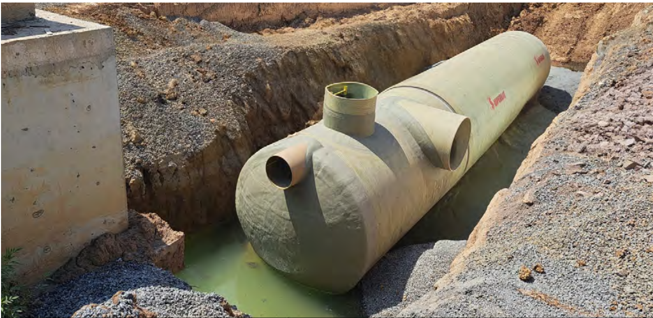
2 Türkiye - Ömerli Kasaba Houses Storage Tank Project DN3000
