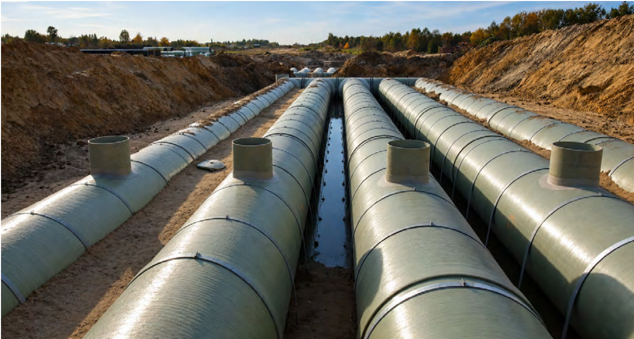
6 Poland - Construction of A1 Motorway Project DN3000
