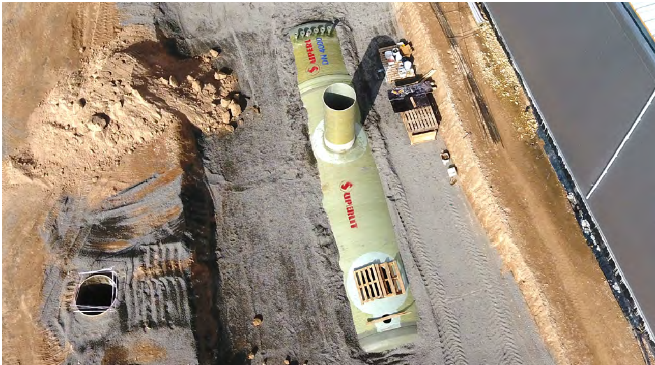
7 Türkiye - Serabiz Sedimentation Tank Project DN4000
